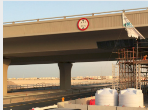
Bridge strengthening Bridge N29, Qatar
