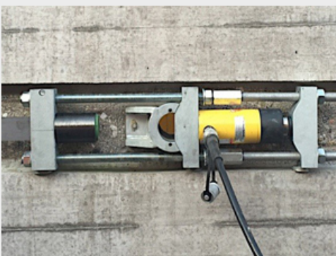
Step 4: Post-tensioning the CFRP plate
